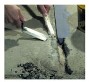
Joint sides should be clean and dry. Spalled joints should be repaired initially using Watco Concrex. (For best results use Watco Back Up Rod to reduce deeper joints to the desired depth.)
