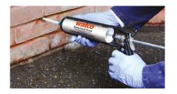
Watco Damp Proof Course is a water repellent, highly concentrated silicone cream packed into a 310ml foil cartridge. It is a thoroughly effective way of treating rising damp while avoiding specialist injection systems.
