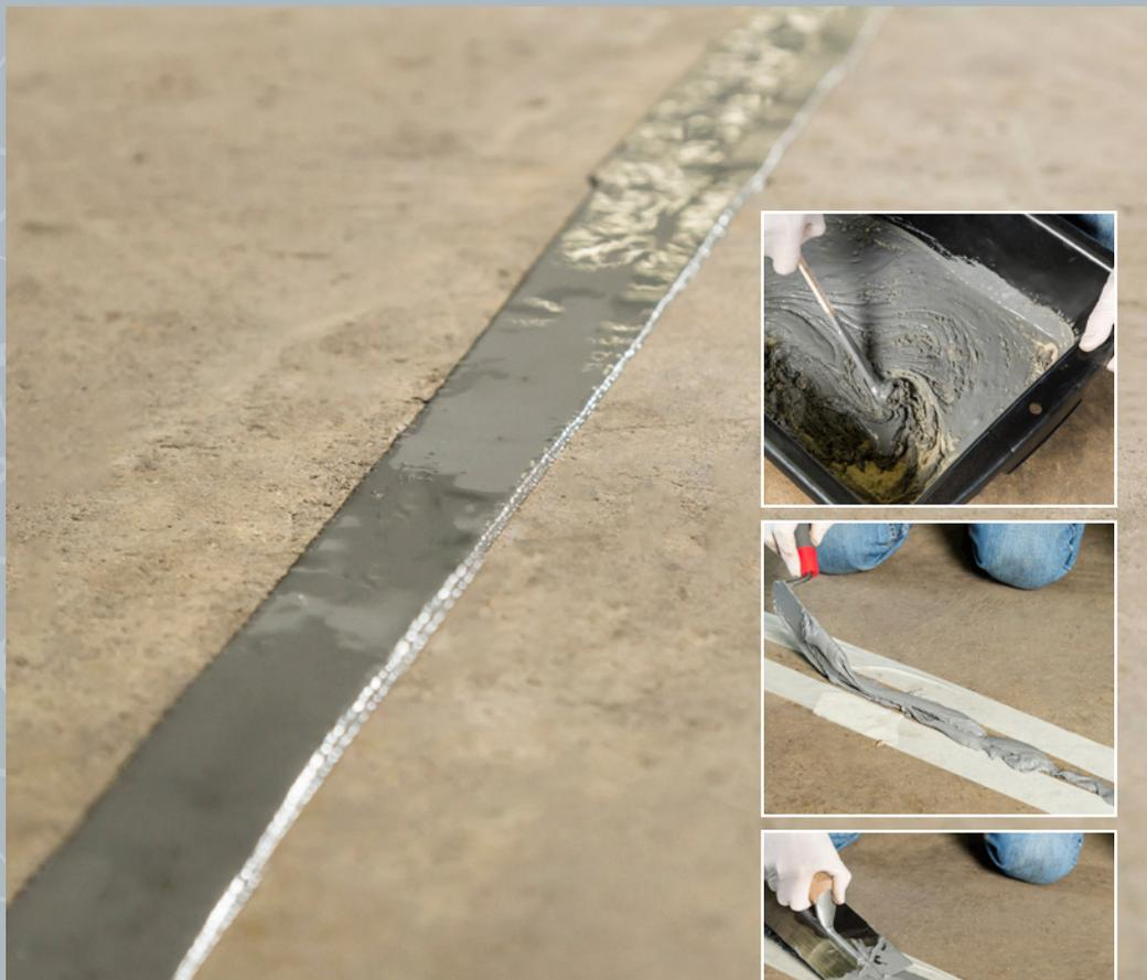
Most concrete floors include expansion or movement joints which are generally filled with a flexible filler. The concrete joint edges can break away with wear and tear and deteriorate quickly as fork lifts and trolleys pass over them. Traditional repairs require the joint edges to be reformed with mortar and the joint filled with expansion materials, a time consuming two stage process.
