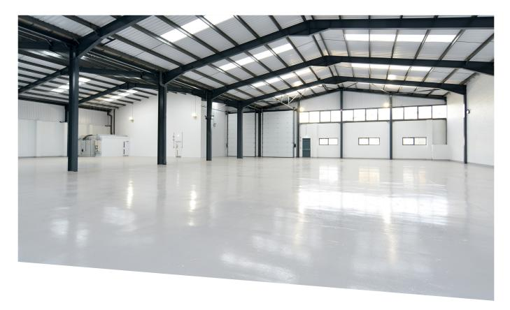
Powerfloated floors are a more common type of industrial floor as they are extremely hard, smooth and easy to maintain which makes them ideal for heavy traffic areas such as warehouses and showrooms. The finish is achieved by working freshly poured concrete and then power trowelling it to a smooth finish using a machine with rotating blades to produce a polished, dense surface.
